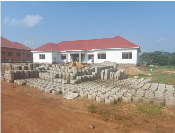
new block nearing completion
