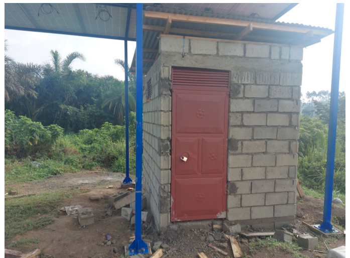
completed solar pump house for water
