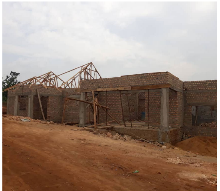
dorm and training blocks under construction
