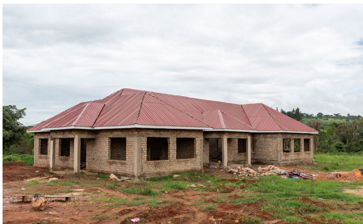
one of the new blocks still under construction
