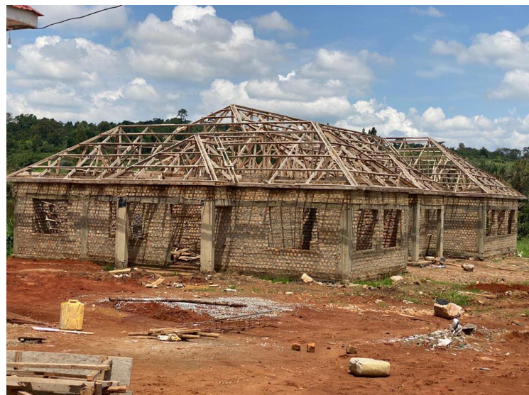
administration block still under construction
